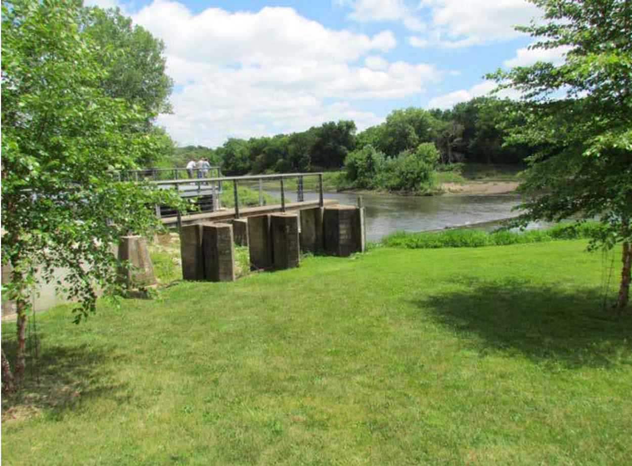
Photo of Sluice Gates
