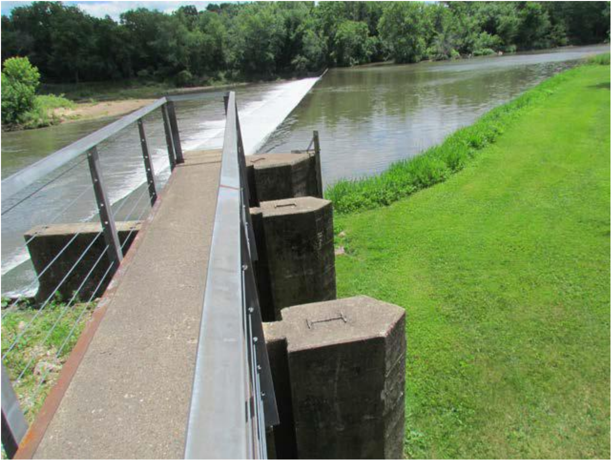
Photo of catwalk above sluice gates showing excavation required to reconnect upstream pool to gates.
